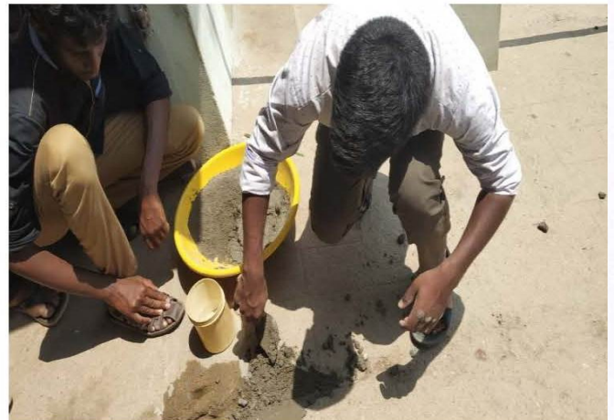
NSS volunteers plastering cement in High School
