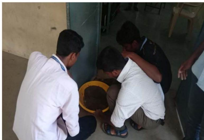
NSS volunteers plastering cement in High School
